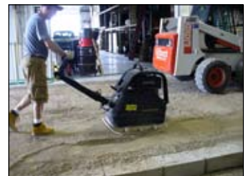
Final compaction
